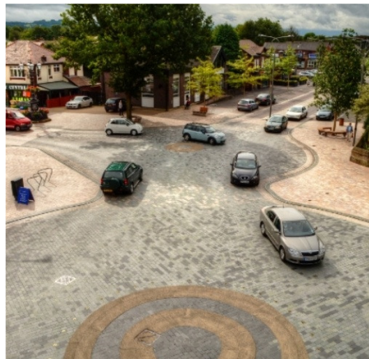
Figure 2: Case Study –Shared Space, Poynton, Cheshire, by Hamilton-Baillie Associates
