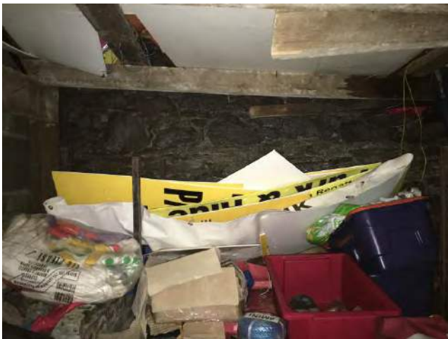
Typical internal view
