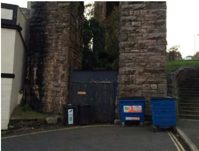
Existing sheds opposite
