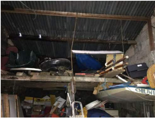
Typical internal view
