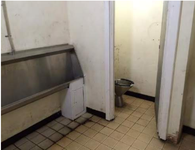
Internal view of male toilets
