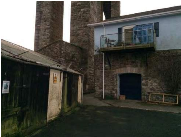
Access to sheds and adjacent Bollard House dwelling
