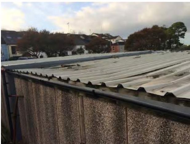
Existing roof and eaves
