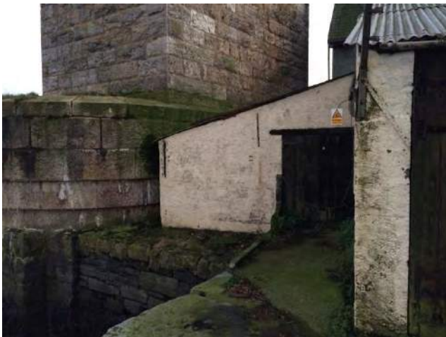
Additional accommodation adjacent to railway bridge column
