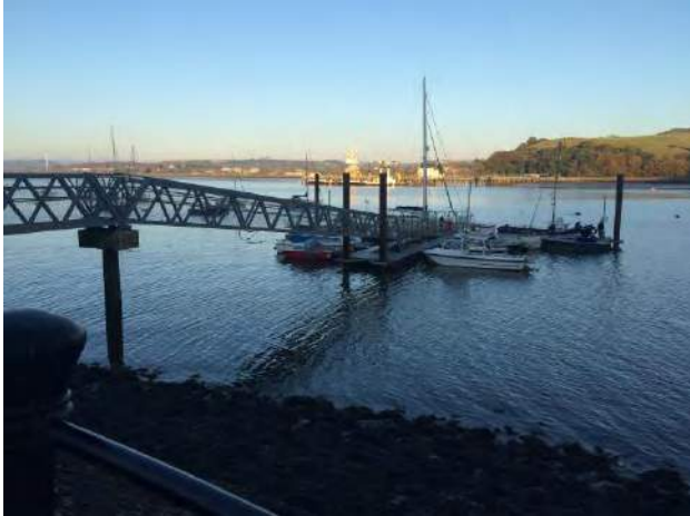
View of pontoon from car park
