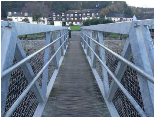
View towards car park
