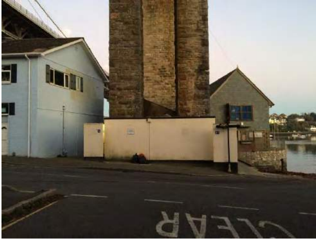
Front view of the existing toilets
