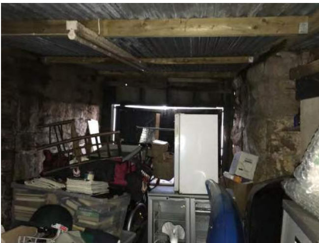
View inside shed
