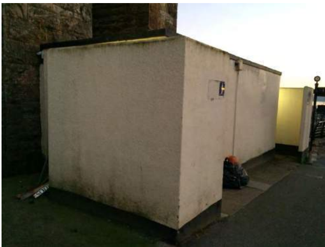
Side view of the existing toilets
