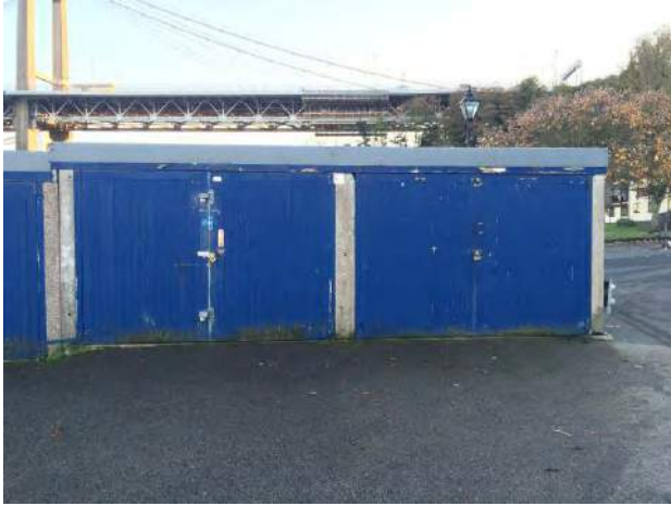
Typical external view
