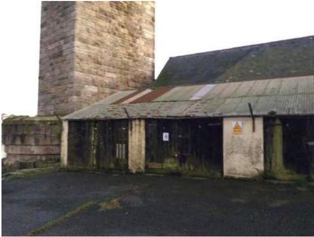
Front view of Ash Wharf Sheds
