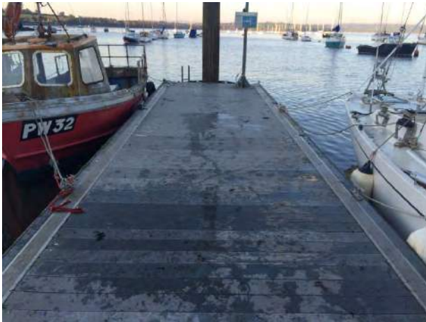
Typical view of pontoon
