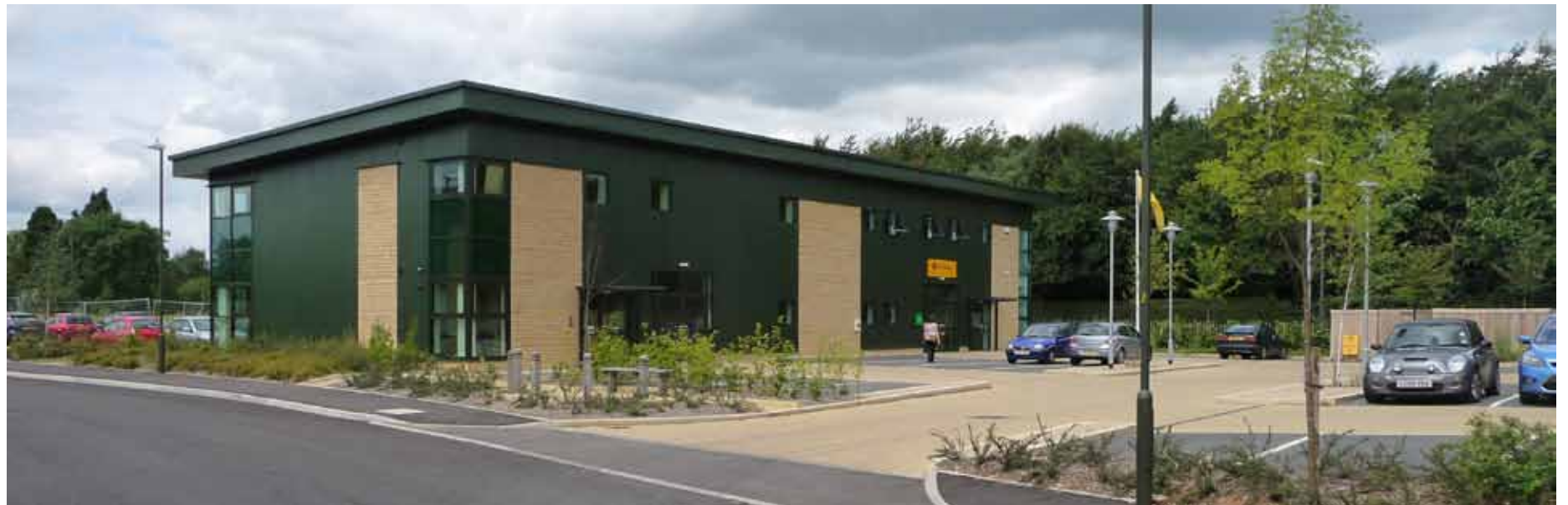
Two storey units front onto adjacent parking, Cotswold Business Village
