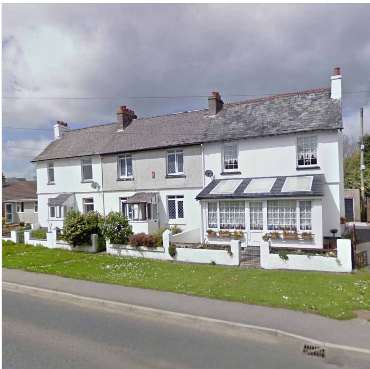
Setback terraces (Pinkhams Cottages) with landscaped verges along the A388, Carkeel
