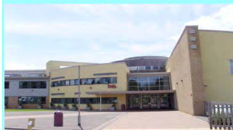
Above: Isca College Exeter; Three Schwegler nestboxes have been fitted to the high brick wall to encourage Swifts to nest there. Photo © Emily Statworthy, Devon Wildlife Trust
