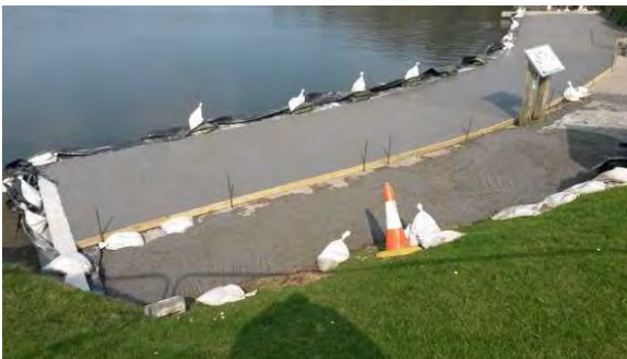
Figure 3. The repaired pavement. Copyright © 2016 Spalding Associates (Environmental) Ltd.
