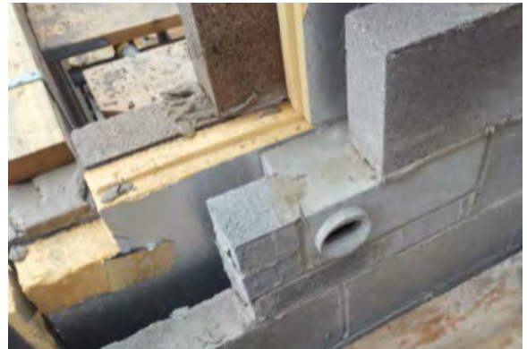
Figure 4. Block wall installation with integrated box
