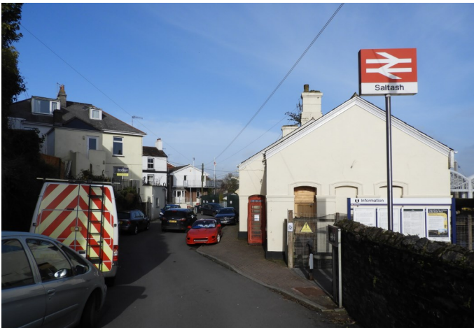
Photo 53: Saltash Railway Station Building. Timely revival has matched service improvements in Spring 2019.
