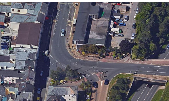
Photo 47 Above: Simons Corner candidate transition zone from national road network to local Fore Street.
