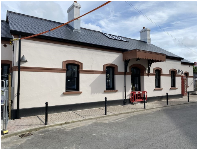
Photo 40: Railway Station Building: a major opportunity for enhancement now nearing completion.
