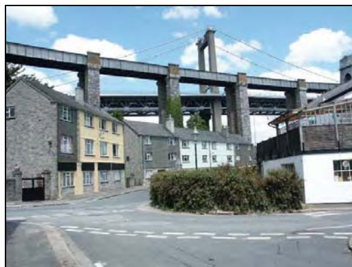
The columns of Brunel's railway bridge rising above the Waterside area
