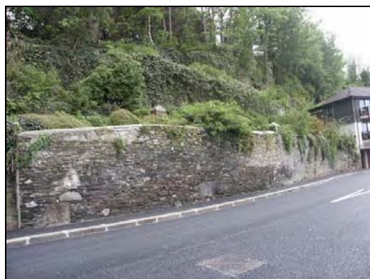
Walls used by the Victorian engineers to sheer up the cliff adjacent to the quarry
