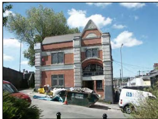
The Drill Hall
