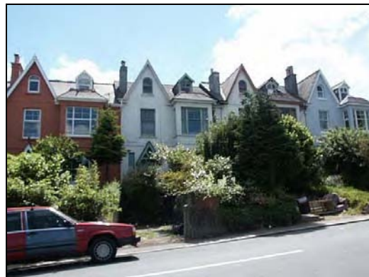
Conservation status could help protect against the loss of character through inappropriate alterations and demolition
