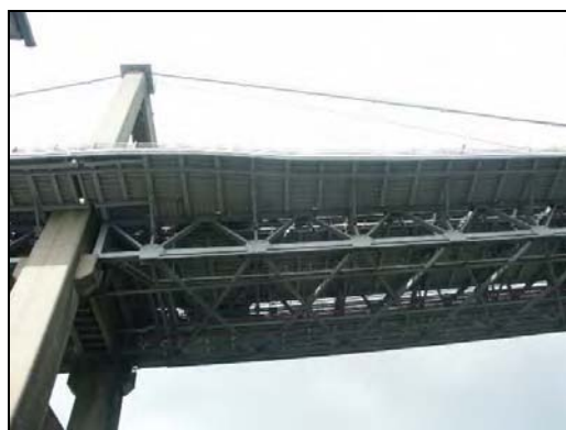
The road bridge, built in 1961, and officially opened the following year
