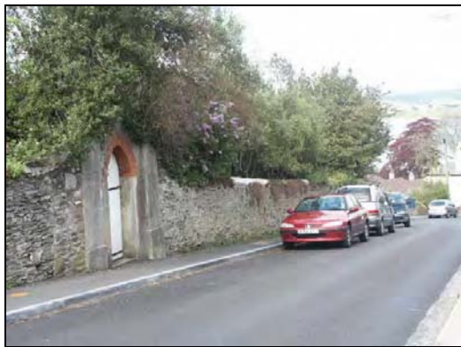
These charming walls that contribute so much to the streetscape are currently unprotected
