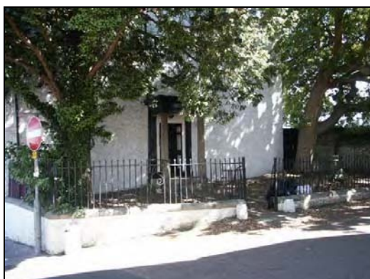
The western porch of Duncan House
