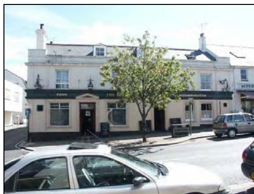
The Brunel Inn, Fore Street – the façade still retains many Victorian details
