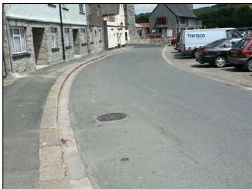
The road surface on Tamar Street could be softened
