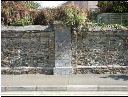
Original walls on the Port View estate
