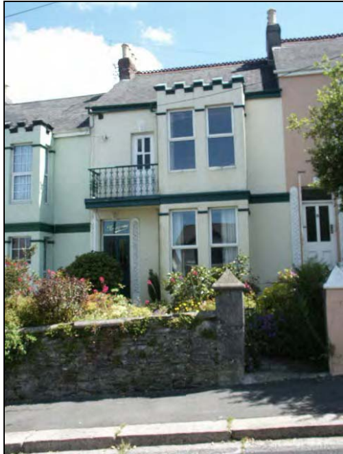
Terraced house on Home Park Road with crenellations and balcony
