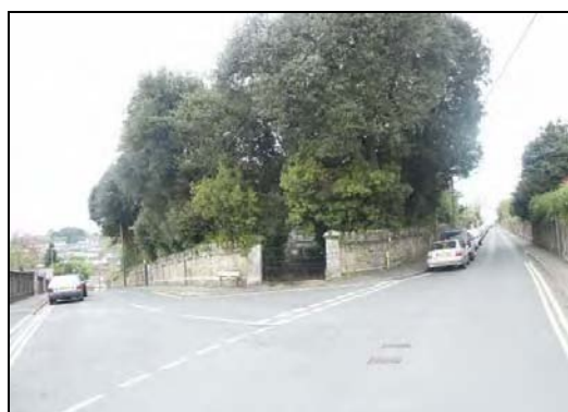
Garden walls could be lost if left unprotected
