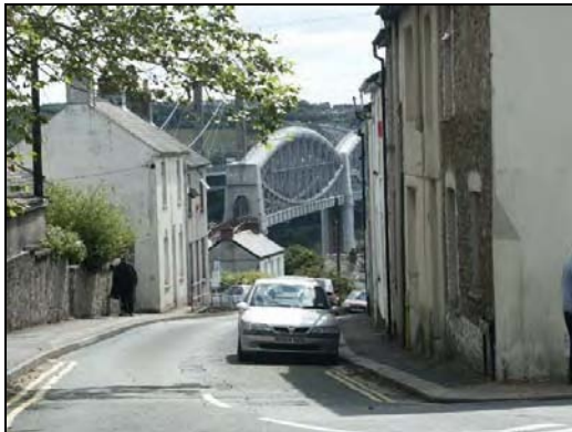
View of the railway bridge from Albert Road
