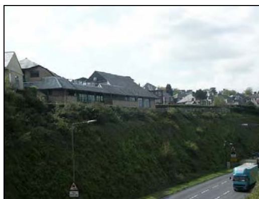
The engineered road leading from the road bridge into the Saltash Tunnel
