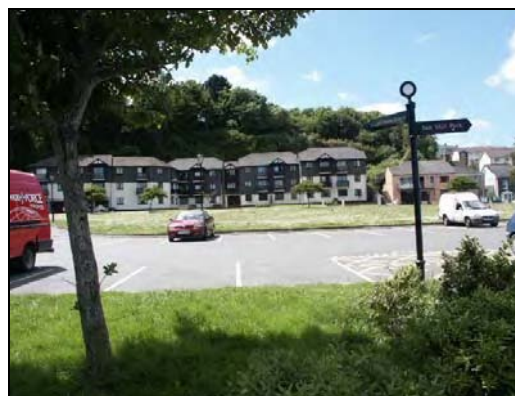
Further work is required in the Jubilee Green and Brunel Green area
