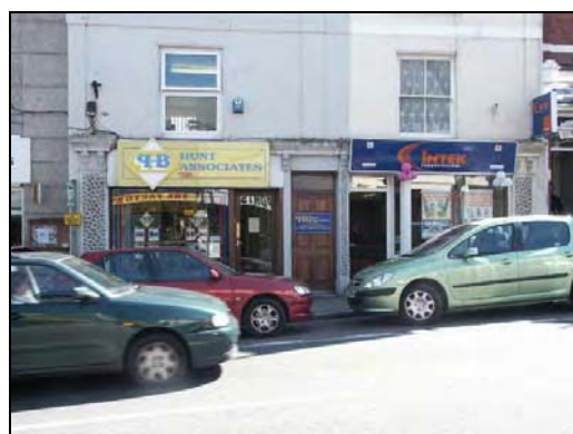
Poor quality shopfronts on Fore Street overlying historical detailing
