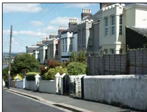
Terraced housing on Home Park Road
