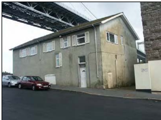
From the road this building on Ashtor Wharf appears to be modern
