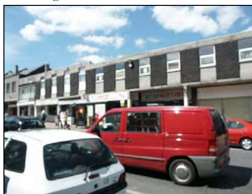
These poorly designed shops in Fore Street do not reflect the quality found elsewhere in the town
