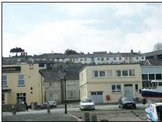
The Boy's Club appears tired and in need of maintenance
