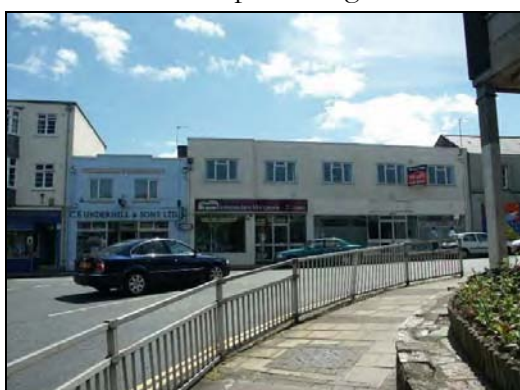
Some of the shops on Fore Street are presently empty
