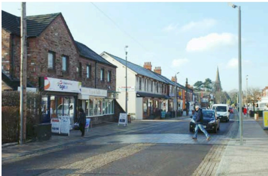
Figure 6.4 Courtesy crossing, Poynton
