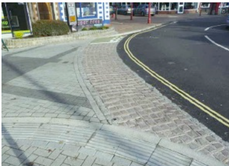
Figure 6.2 Example of a shared space gateway feature
