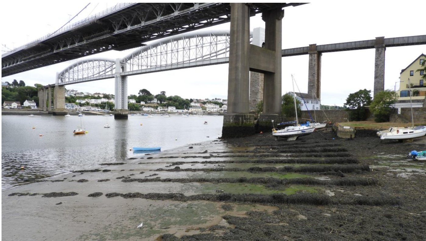
Above, Looking SE at foot of road bridge is former WW2 Landing Ship Repair staithes, a heritage feature.
