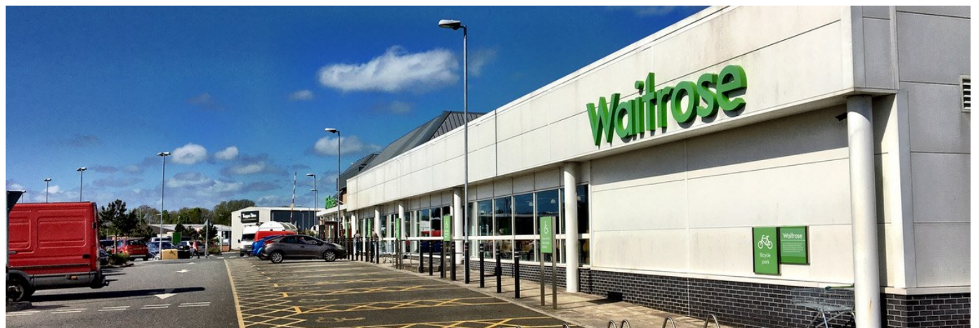
Photo 32: Waitrose at Carkeel, outside the town centre but attracting many shoppers from a wide catchment.
