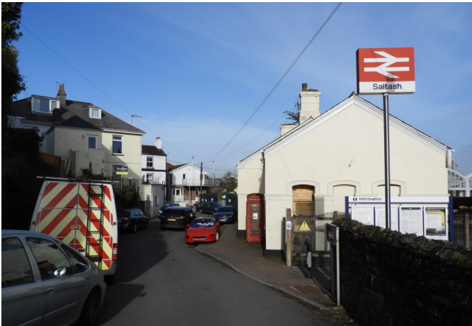
Photo 53: Saltash Railway Station Building. Timely revival will match service improvements introduced in Spring 2019.
